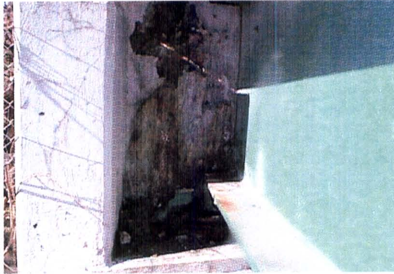
SPALL WITH EXPOSED STEEL AT ABUTMENT #2 LEFT SIDE
