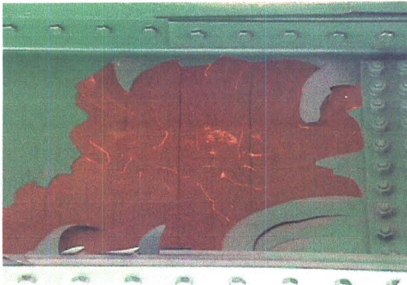
PEELING PAINT BEAM "A AND C"
